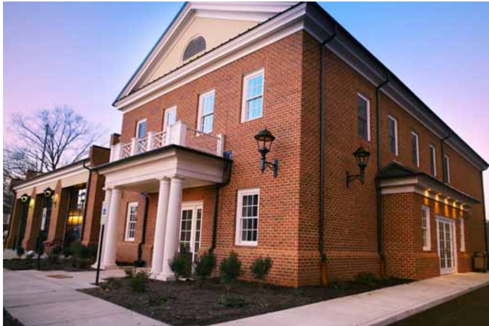
The Palmyra Fire Station is a prime example of the project diversity CMS, Inc. has produced while collaborating with local architectural firms Land Planning & Design and Dalgliesh, Gilpin, Paxton Architects.
